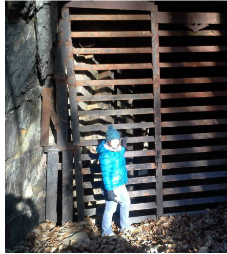
Left: Recently, Craig & Melissa Telesha explored the old York Iron Co. Mine Site at Raab Park. (Mining ended in the 1890s) Grating on this shaft allows a safe habitat for bats. Haunted? Perhaps (Mining is dangerous) Creepy? You bet! Does Melissa have bats in her belfry? Dunno, but I've been accused of it - JDW
